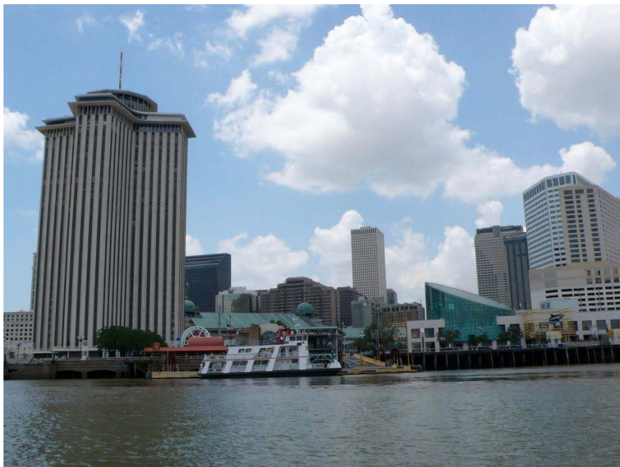
Algier's Ferry, wharves and docks along waterfront at the base of Canal Street
